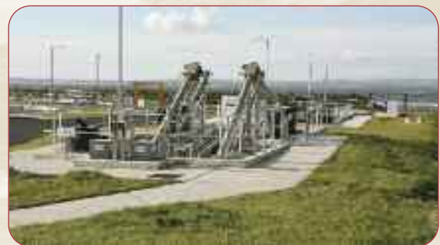
Enniscrone Waste Water Treatment Plant. Photo by Steve Rogers.
