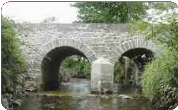
Leekfield Bridge, Skreen.
