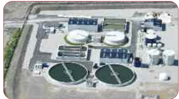
Sligo Wastewater Treatment Works.
