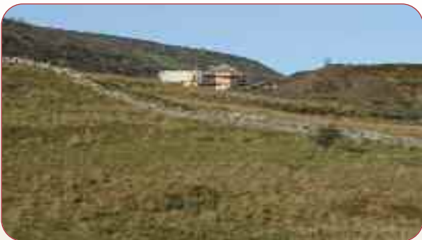
Site works at Keash GWS Site.
