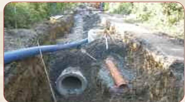
Pipelaying during Construction of Teesan/Lisnalurg contract.
