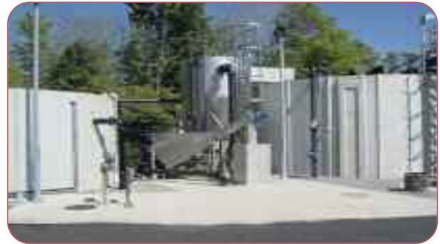
Coolaney Waste Water Treatment Plant.
