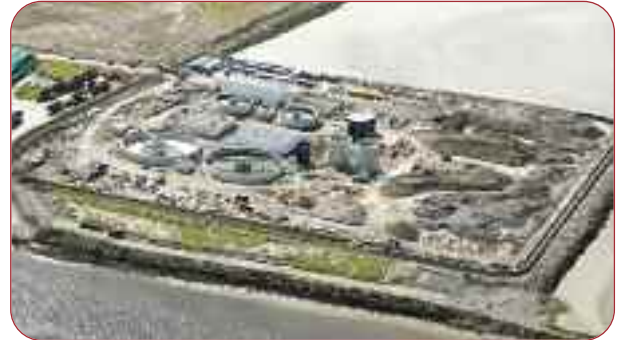
New Wastewater Treatment Works During Construction.
