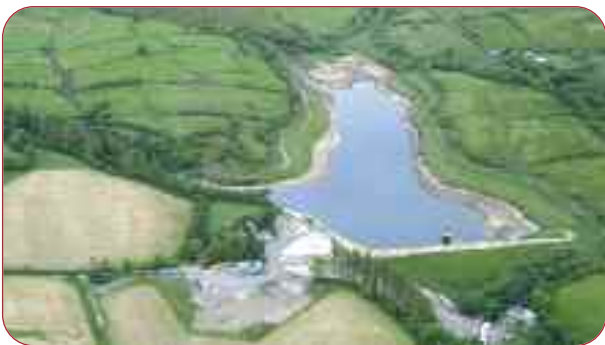
Kilsellagh Reservoir. (During Kilsellagh Dam Modification Contract)
